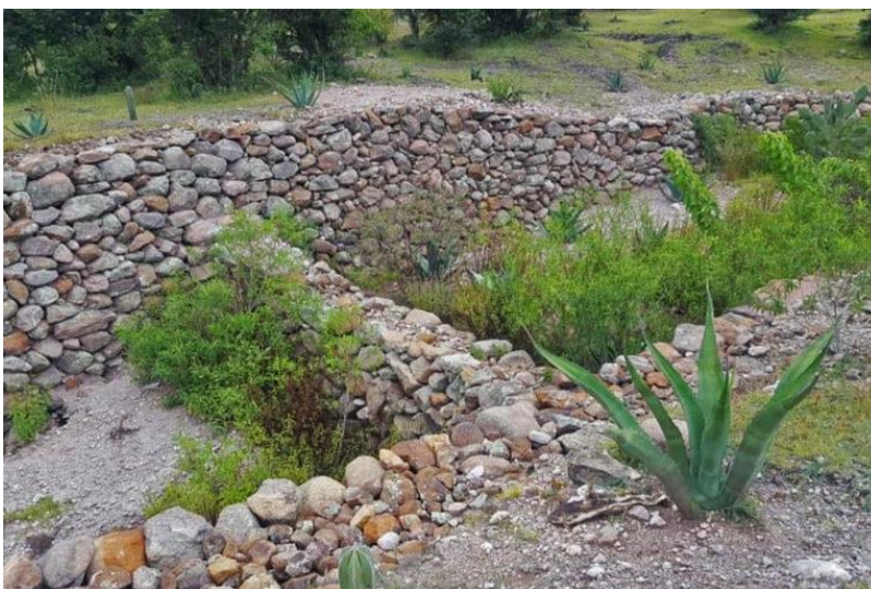
In 2019 and 2020, members of the Ejido Los Toriles community — aided by a community, management, soil recovery and reforestation specialist — built stone barriers, known as gaviones. These barriers will stem runoff from the watershed after heavy rain, allowing earth and vegetation to start accumulating in the gavion, resulting in soil recuperation. As the photo shows, agaves are also planted in strategic places to fix the soil in place more firmly. Image courtesy of Alejandro Vasconcelos.
